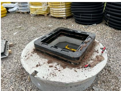
TORiser can be laid using standard sand & cement bedding mortar or if specified polymer modified bedding mortar.
