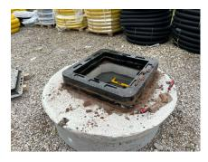
TORiser can be laid using standard sand & cement bedding mortar or if specified polymer modified bedding mortar.
